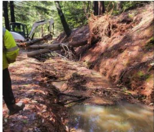
**This photo displays the amount of captured water as a result of rainfall and run-off, in addition to the impacts of the hillside when a tree collapses and exposes the root ball.**
