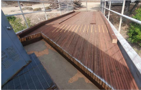
Station 8 Replacement Wood Decking
