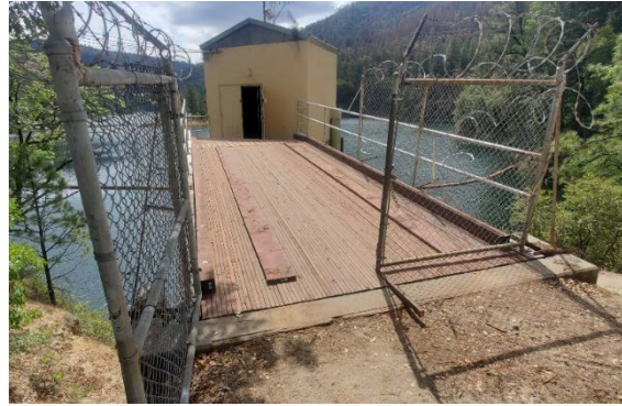
Station 8 Replacement Wood Decking
