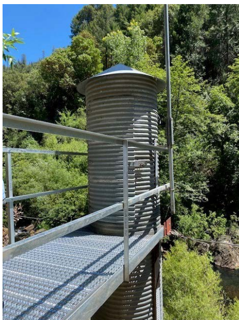
SF-17 Replacement Metal Access Platform
