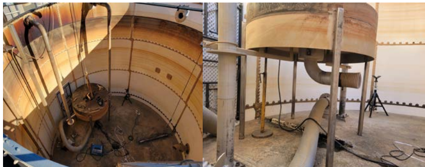
A homogenization tank is mainly intended to stabilize flow and the waste load.
