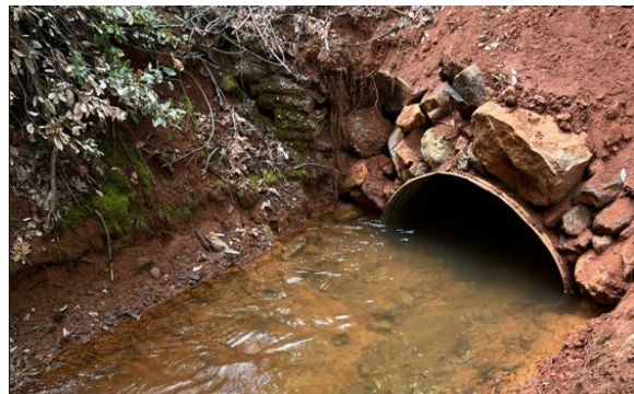
Water flowing after culvert repair
