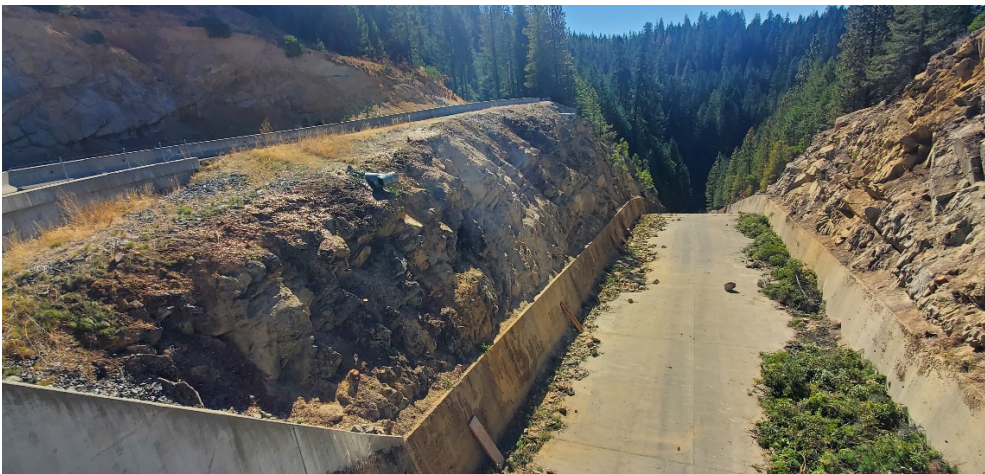
Sly Creek Spillway after scaling of embankments.
