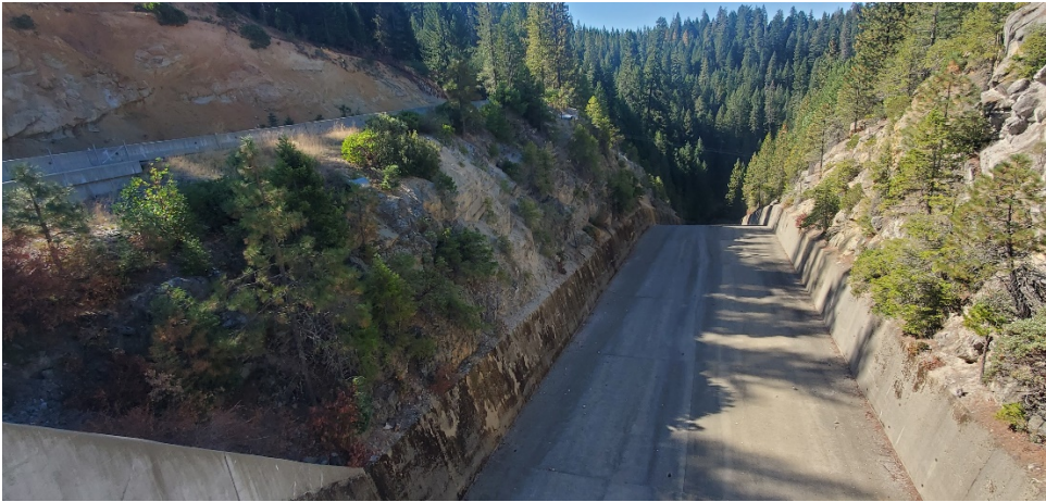
Sly Creek Spillway before scaling of embankments.
