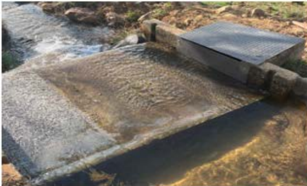
Concrete work performed by SFWPA crew in the North Ditch (Pincrest between Upper Palermo and Drescher Tract area)
