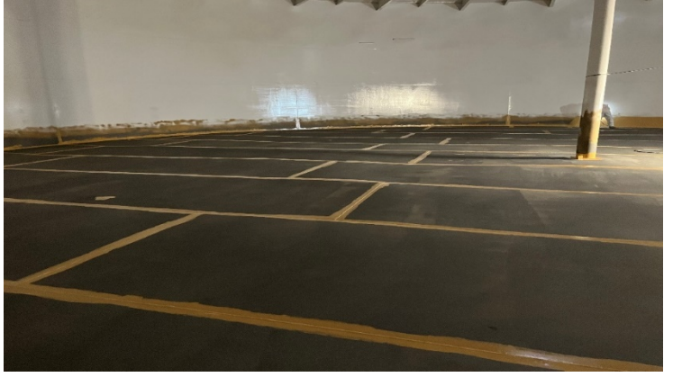
Welded Seam Protection:
