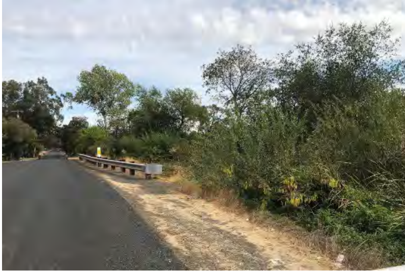
Photo 1. Bridge crossing over seasonal channel between Railroad Avenue and Melvina Avenue. All planned construction will take place within the roadway right-of-way.
