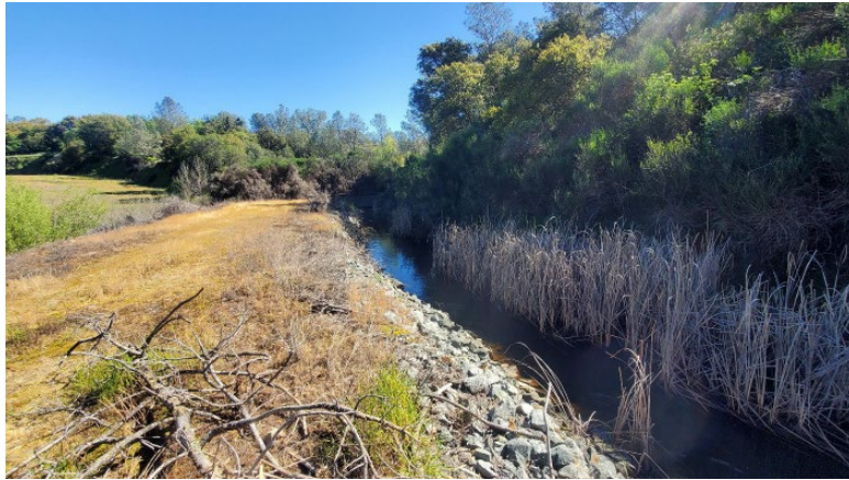
Vegetation growing in SF-25 earthen intake structure, view downstream
