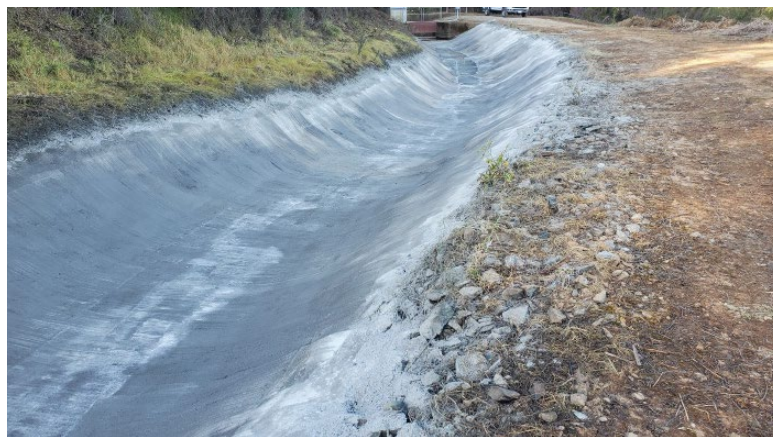
Newly applied shotcrete at SF-25 intake structure, view downstream
