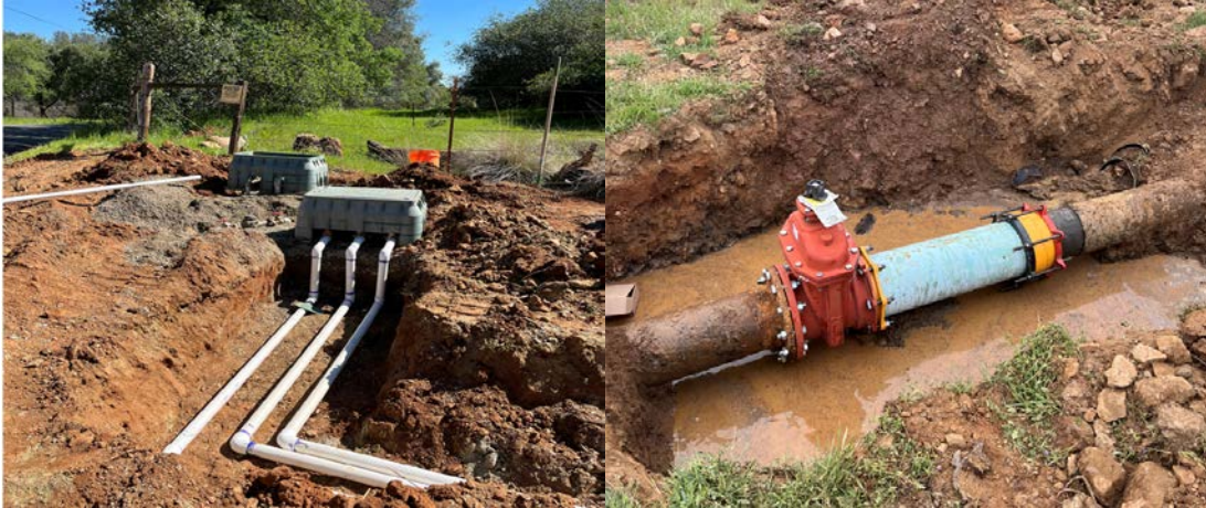
Dunstone Valve Project
