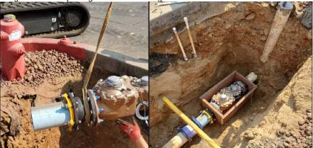
This assembly has both "high" flow and "low" flow measurement capability.
